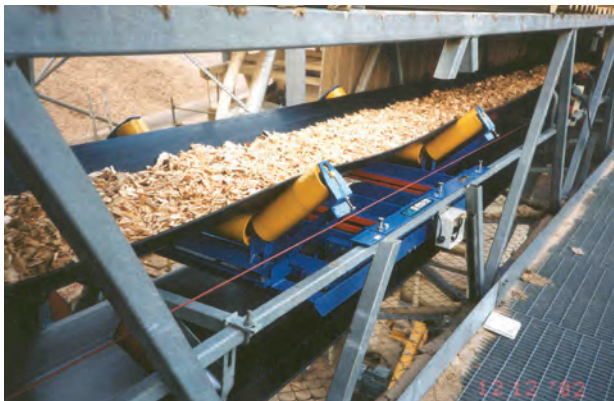
Wood Chip Conveyor
