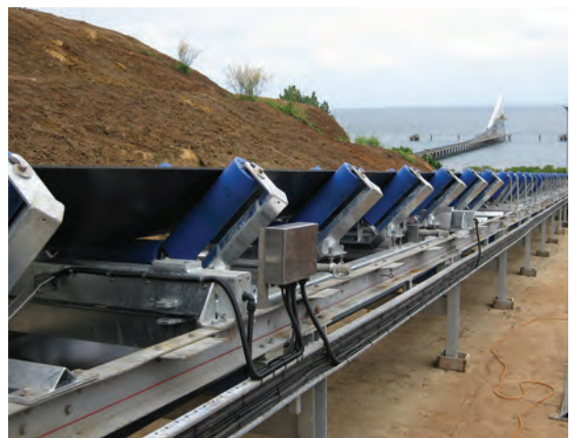
Four Idler Belt Weigher on wood chip ship loading conveyor
