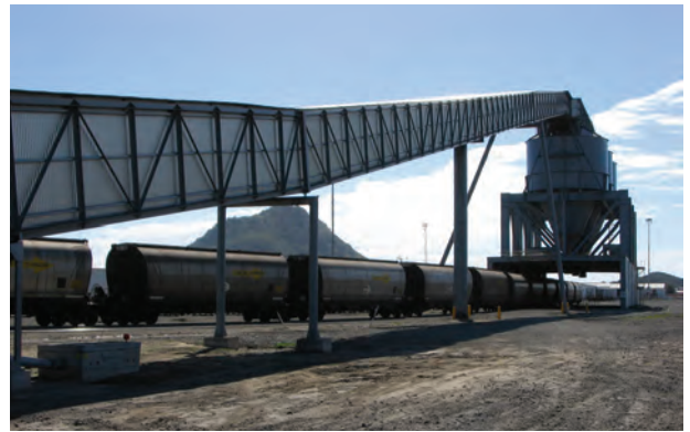
Enclosed installation on train loading coal conveyor
