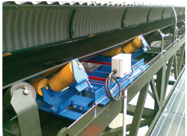
New B152 installation on coal conveyor
