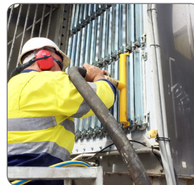
Dust Collector Servicing
