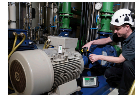
Industry: LASER-EQUILIGN2 always ensures professional alignment of your machines thanks to single laser technology
