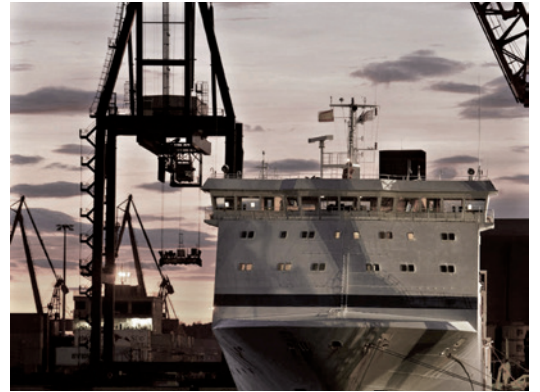
Harbour crane for ship loading.
