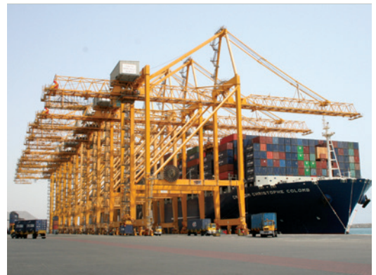
Ship to shore cranes.
