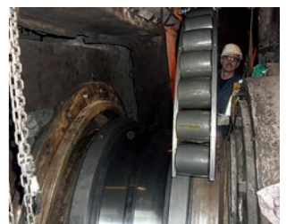
Installing an FAG split spherical roller bearing in a steel converter
